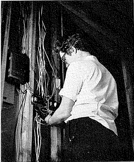
Complex wiring arrangement in house is its owner's pride. One switch operates 13 lights.
